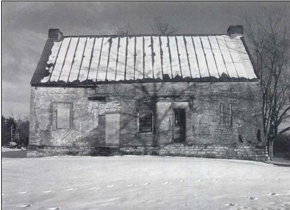
The original main facade of the Jan van Hoesen house has been altered, but its symmetrical arrangement can still be discerned
